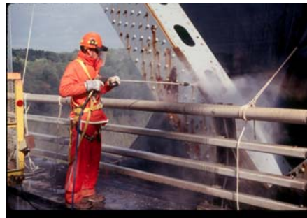
-SSPC-SP12,WJ4: Pressure wash 4,000psi 0° Turbo tip
